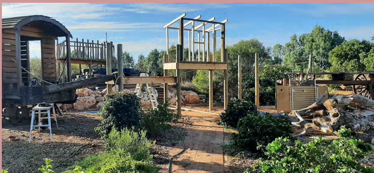
Under construction; Mr Shaw's latest project is connecting the train to the camel cart with a bridge.
